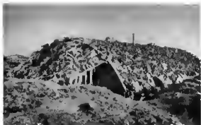
Figure 53. Here is a quonset hut blended into the terrain by a combination of digging in, texturing, and covering with a net.
